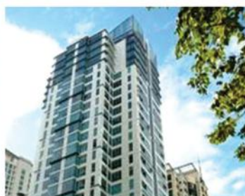
Crescent Park The Fort, BGC - 28 Storeys
