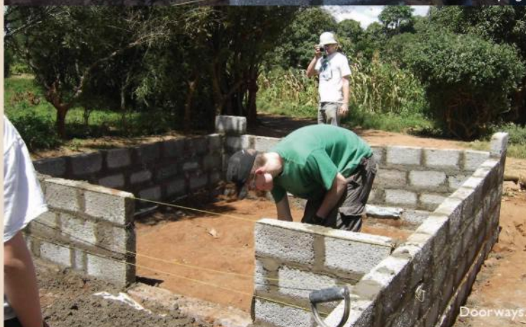
Corners ready for brick-laying.
