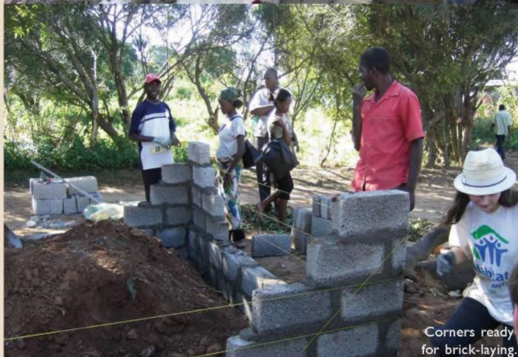
Laying the first layer of the foundation.
