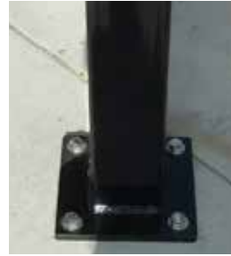
External Anchor Bolts At Finish Grade
