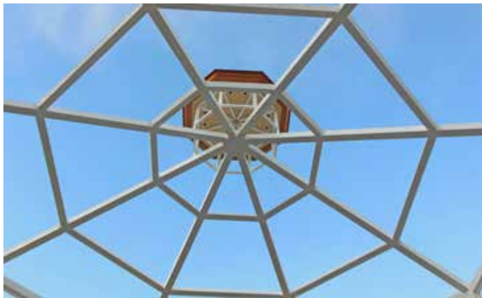
Frame complete and ready for roofing
