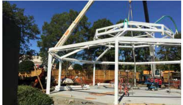
No field welding required during erection
