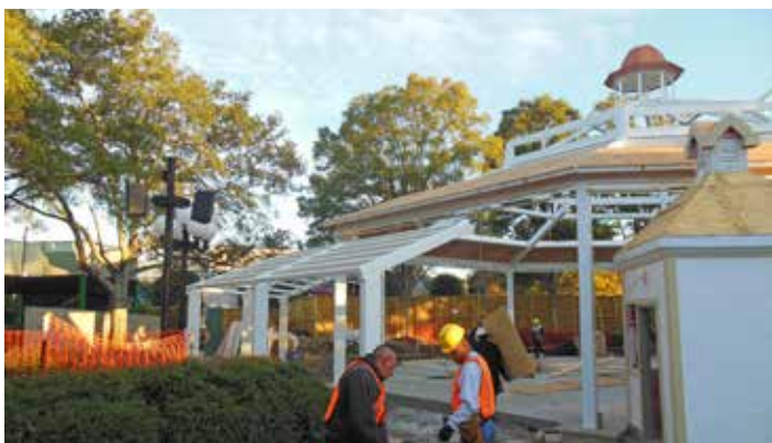
Installation of metal roofing panels
