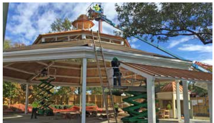
Installation of metal roofing panels
