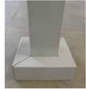
External Anchor Bolts With Cover
