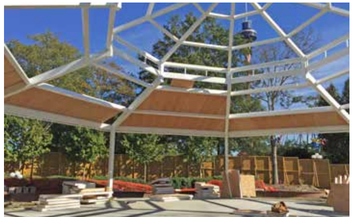
Supporting roof deck is installed
