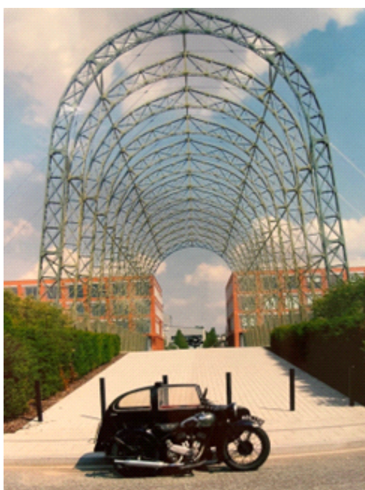
Tricia & Ian Woodford's 1936 Royal Enfield Model K, 976cc, with 1911 portable airship shed structure re- erected thanks to Farnborough Air Sciences Trust (FAST), at the same spot as the original installation.
