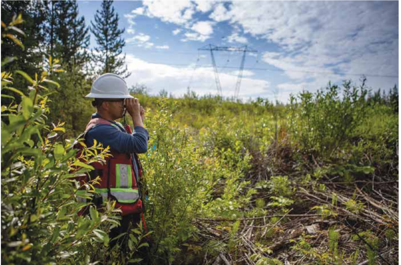
Crews with Kintera, a B.C.-based natural resource company, flag roads and mark GPS points west of Prince George in advance of major construction on the North Coast Transmission Line.
