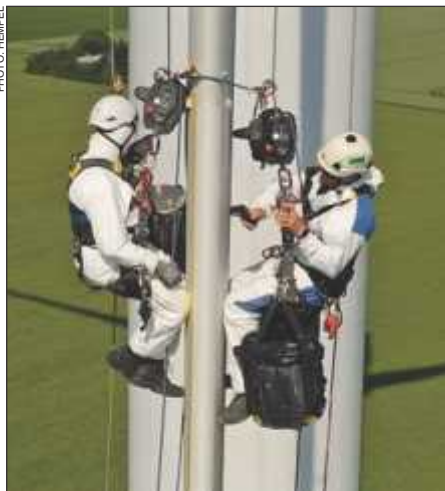
Hempablade Edge 171 is one of the simplest LEP solutions on the market to apply, yet able to withstand the toughest environmental conditions.
