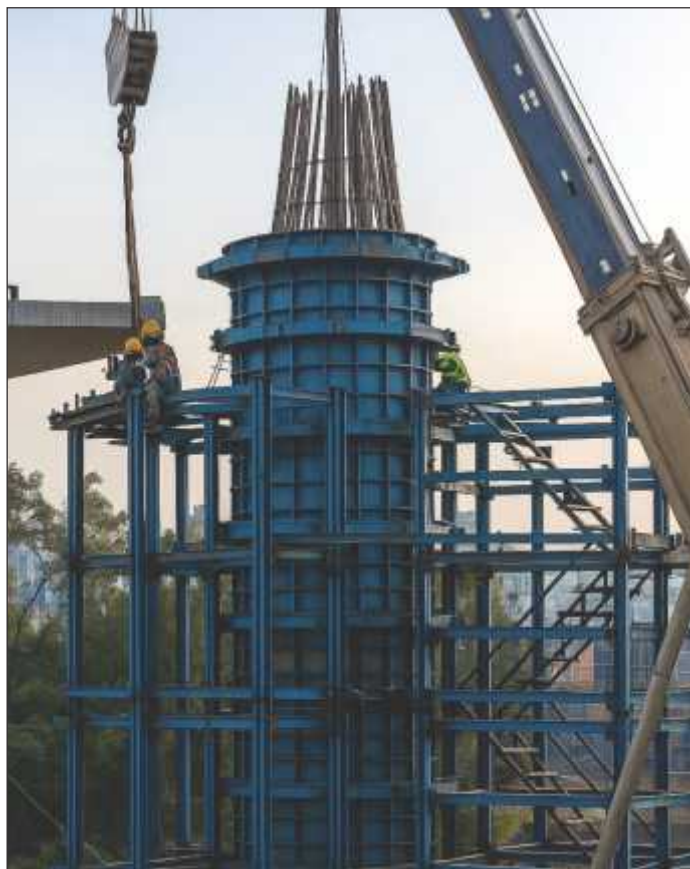
Ringlock systems are modular by design. Components fit together through fixed connection points, reducing the need for complex alignment during installation.
