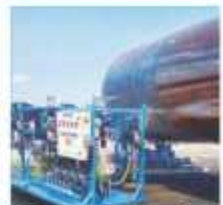
External Automatic Pipe Coating
