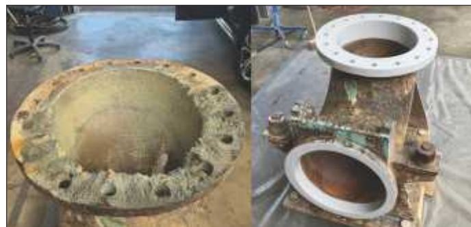
Original geometry of flange restored with Belzona 1000 Series solutions.
