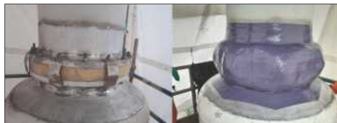
SF 6 leak successfully sealed with Belzona SF6-FIX.
