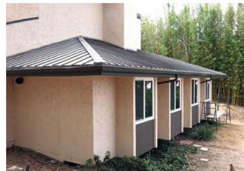
New windows that will provide firefighters views from nearly the top of Mt. Soledad at Fire Station 16.
