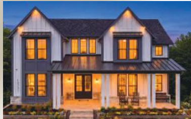
Production Builder Interior Merchandising of a Model Home: $600,000 to $800,000 DREES CUSTOM HOMES FINALISTS: Drees Custom Homes J.Patrick Homes
