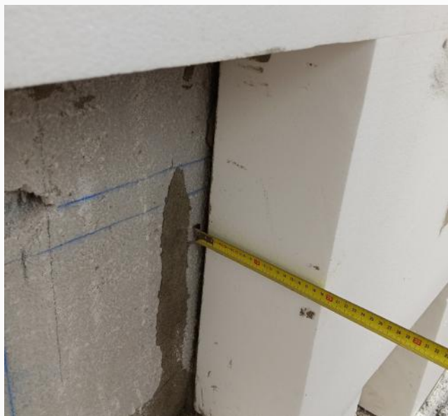
fachada SATE YZ HUB, EPS 180mm
