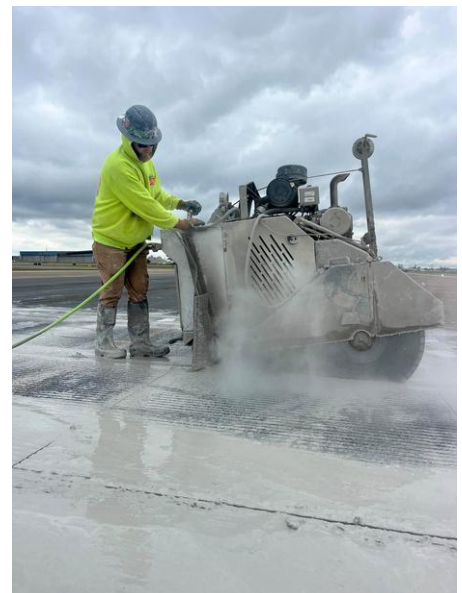
Professional Concrete Cutting & Drilling is based in Columbus, Indiana and currently serves Indiana and neighboring states.
