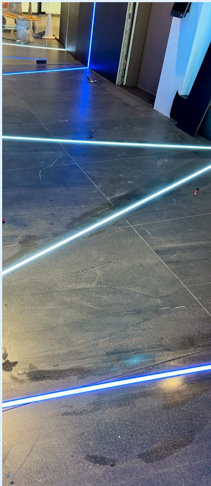
LED light strips are tested after installation to verify alignment and consistency within precision-cut channels in gauged porcelain tile panels.
