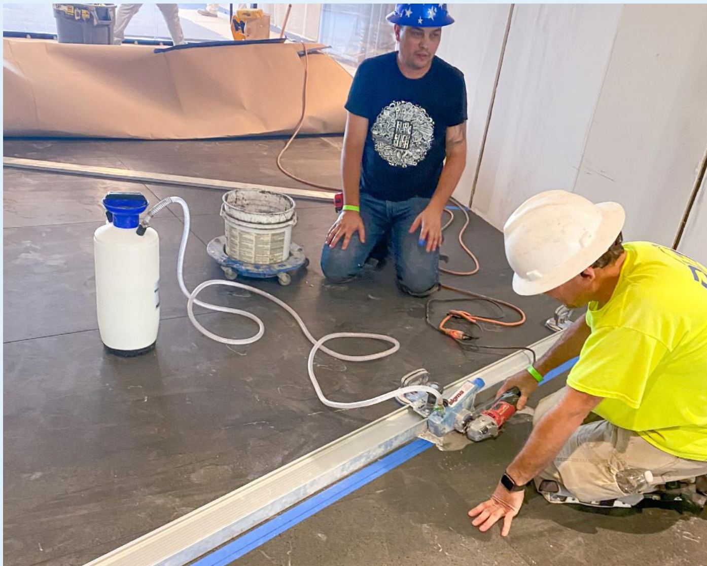
Crew members cut channels for integrated LED light strips using a Sigma Kera Flex adapter on a Kera Cut rail, paired with a Sigma water feed kit for dust control and precision.
