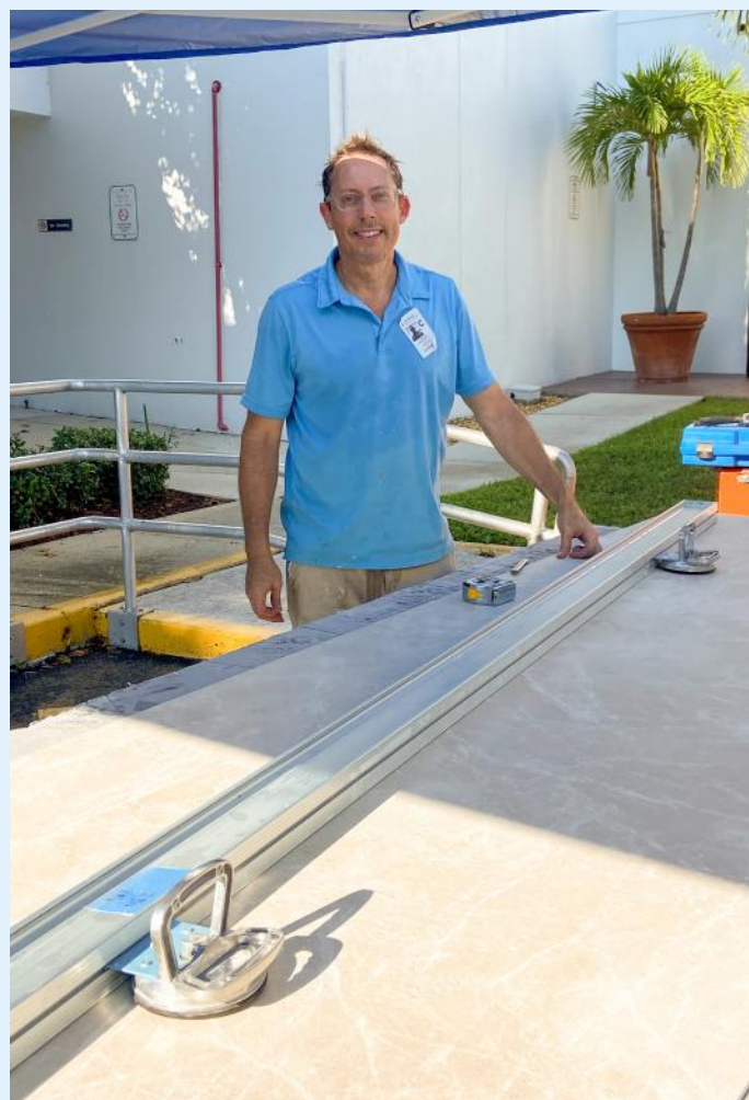
NTCA member Rich Smith, Owner of Porcelain Slab Services, prepares a gauged porcelain tile panel using a Sigma Kera Cut rail system during installation.
