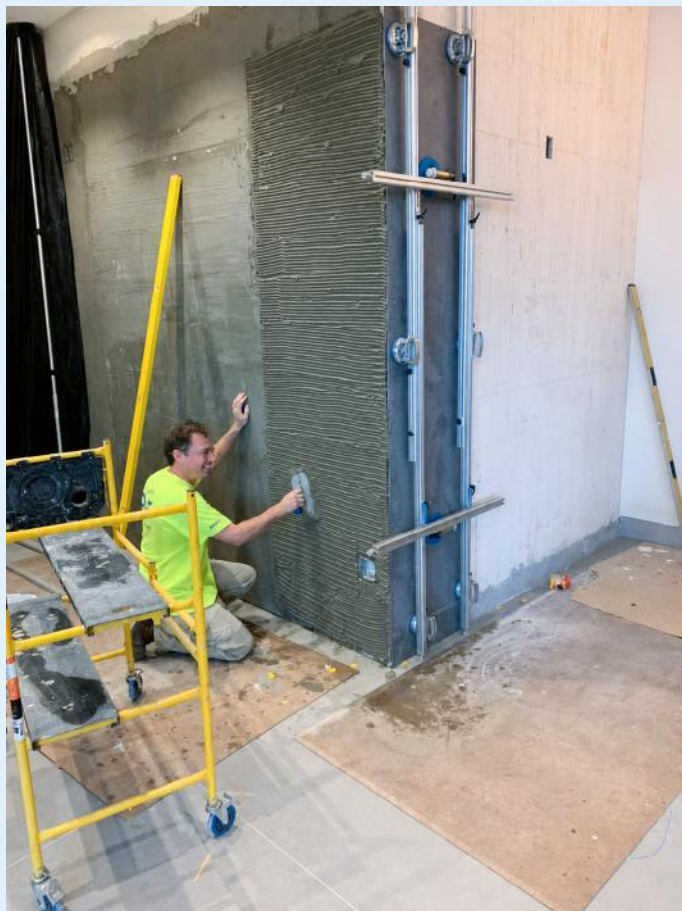
A crew member trowels mortar onto the wall substrate in preparation for installing the next gauged porcelain tile panel.
