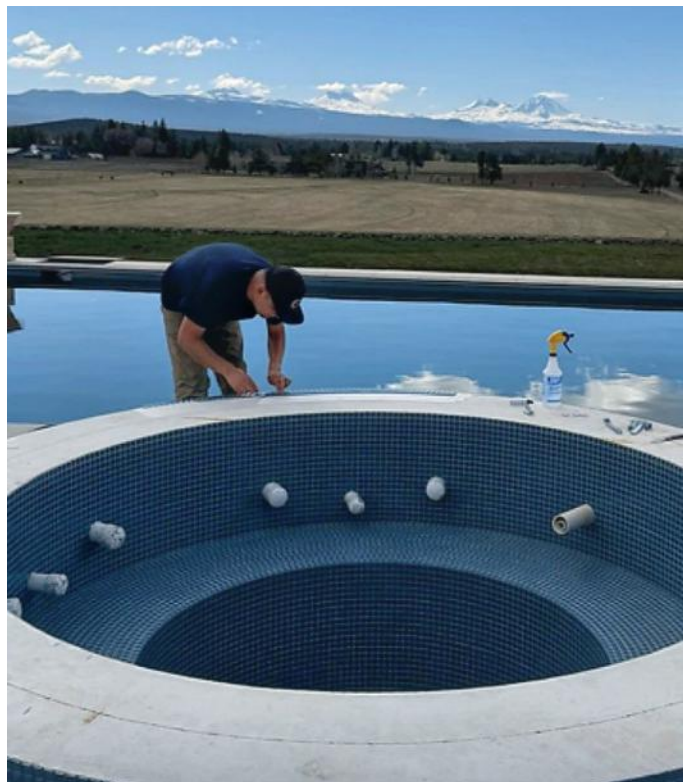
This infinity-edge spa was floated using a rendering mud over gunite. The layout was carefully planned to ensure all the tile finished on full pieces. After the float, the spa was fully waterproofed and finished with glass tile.
