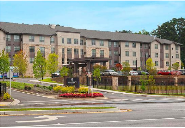
RENAISSANCE AT GARDEN WALK RIVERDALE, GEORGIA
