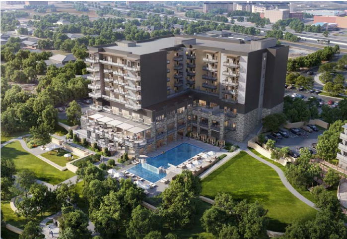
SPRINGHILL SUITES RIVER VILLAGE NEW BRAUNFELS, TEXAS
