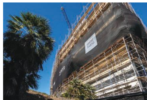
Construction at the old Perry's Cafe building, which developers say will soon connect with their vision for Midway Rising at Pechanga Arena. (Photo by Thomas Murphy/Special to Times of San Diego)
