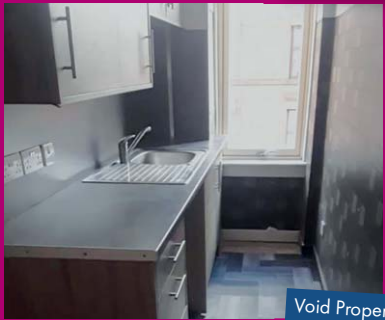
Void Property – Kitchen – Before
