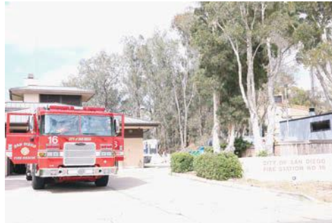
Fire Station 16 is undergoing its first major renovation since opening in 1982. (Photo by Karen Pearlman/Special to Times of San Diego)
