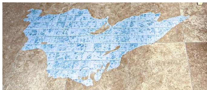
The finished floor.
