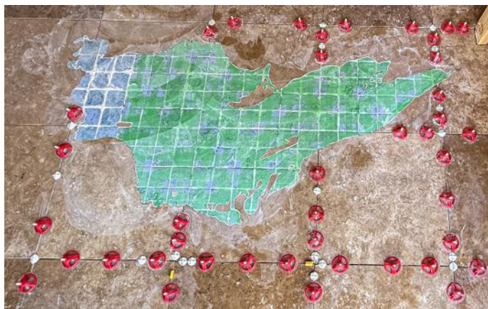
Mosaic installed. Note bond coat oozing through joints under face tape
