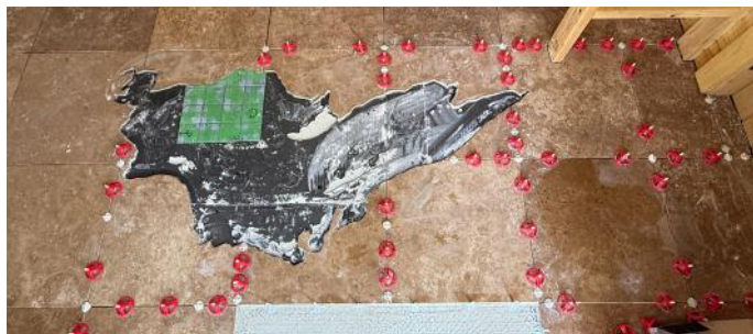
Field tile installed along with wedi backer and mosaic section dry-fit to check height.
