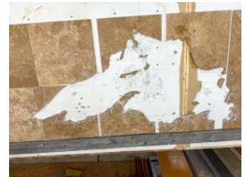
Field tile, fully cut.
