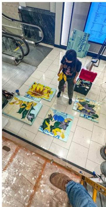
Scaffolding was needed to reach the full 12’ height of the project.
