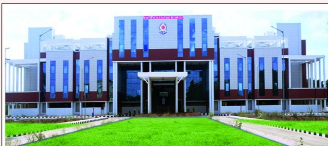
JNTUA ADMINISTRATIVE BUILDING, ANANTHAPURAMU
