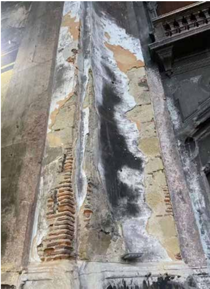
The colours of fire damage are visible on the Church of São Domingos in Lisbon, 67 years after a fire. The vault shows the pink-red tones that signal temperatures above 570 F (300 C). The columns are blackened by soot. Where the outer surface has spalled or chipped away, the undamaged masonry is visible beneath. Tiago Miguel Ferreira
