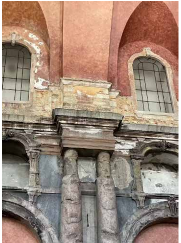
The colours of fire damage are visible on the Church of São Domingos in Lisbon, 67 years after a fire. The vault shows the pink-red tones that signal temperatures above 570 F (300 C). The columns are blackened by soot. Where the outer surface has spalled or chipped away, the undamaged masonry is visible beneath. Tiago Miguel Ferreira
