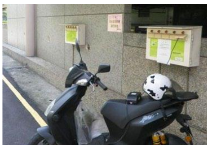
▲ Electric Scooter Charging Station
