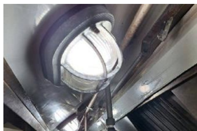
▲ Removing Paint from Shatter-Resistant Light Covers
