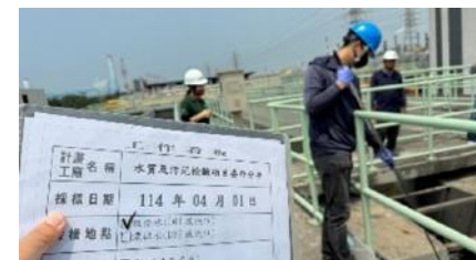
▲ Water Quality Survey at the Water Resources Center
