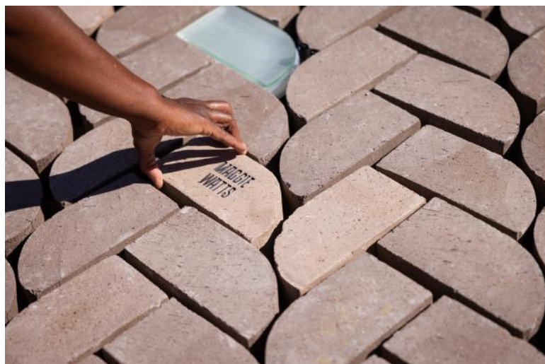
Installation of twelve thousand custom-poured clay bricks comprising the monument's braided pathway.
