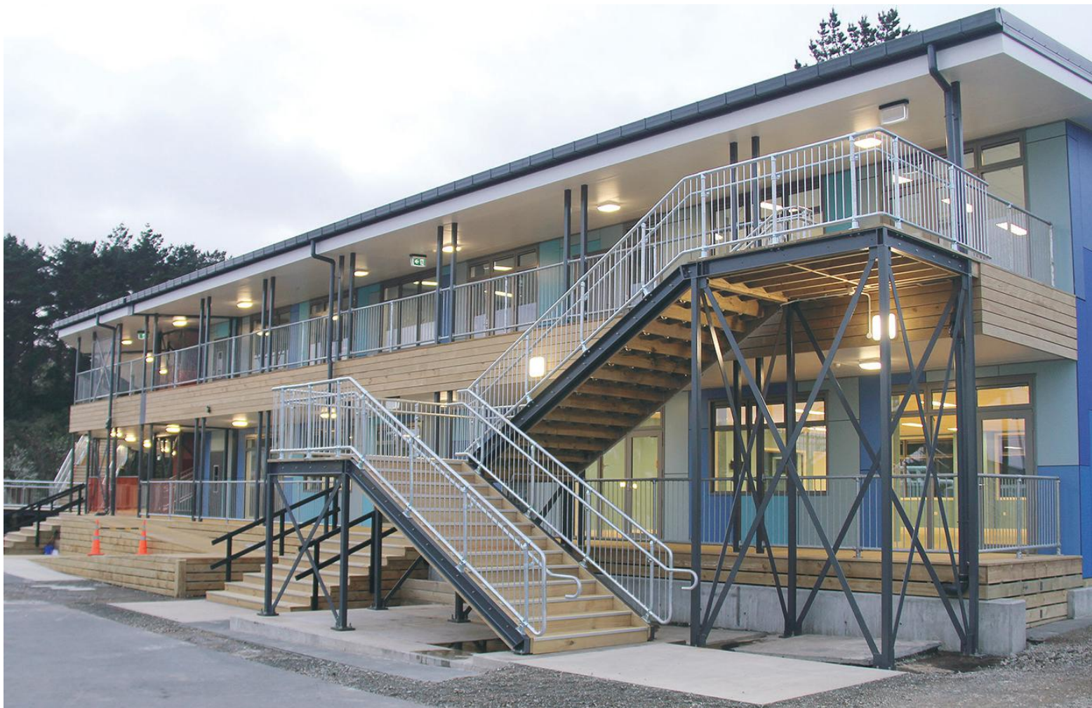
The new $2.3 million classroom block at Newlands Intermediate School, which was blessed on 21 September. Photo: Supplied.
