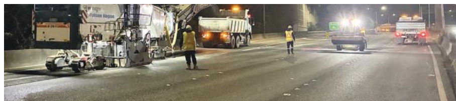
Road resurfacing, which is planned for State Highway 1 next month, taking place. Photo: NZTA/Waka Kotahi.
