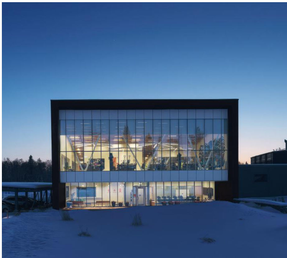
Left: Nordic data centre powered using local hydro-electric power, capitalising on the cooler environment.
