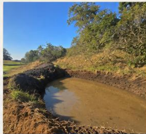
Early stages of the dam taking shape.
