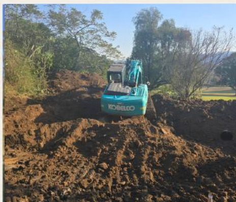
Excavation in progress to shape the new attenuation dam.
