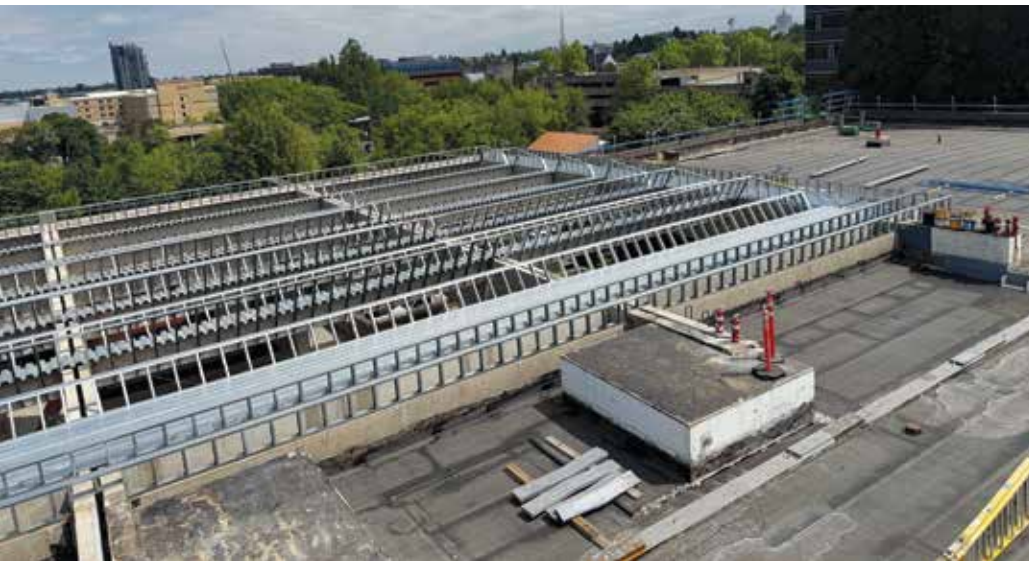
The centerpiece of the Salem Civic Center project is the seismic work. The addition of six reinforced concrete shear walls along the building's exterior.
