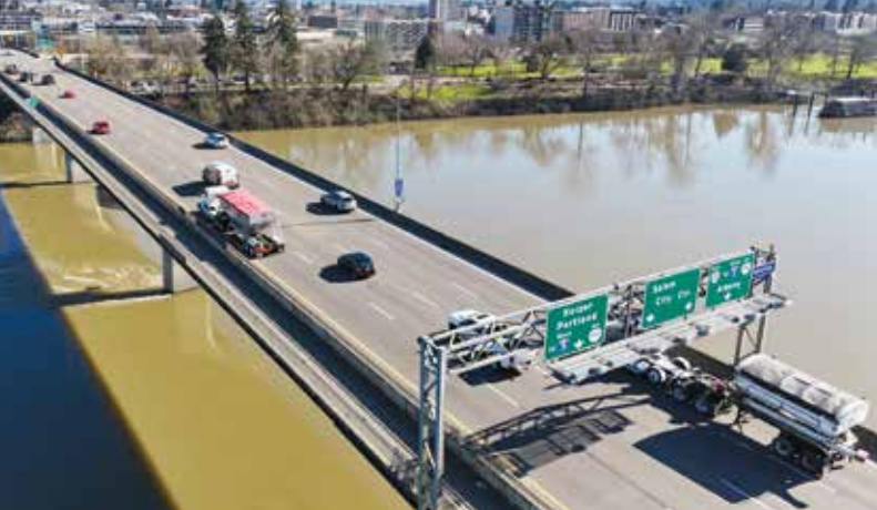
R-22 Eastbound Center Street Bridge to downtown Salem.
