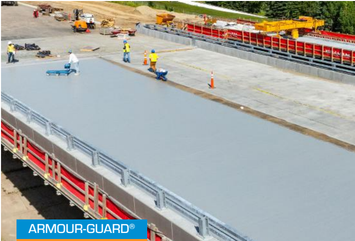
T-17 POLYMER CONCRETE
