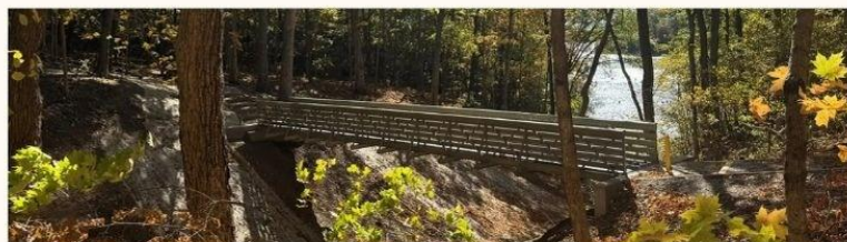
NEW BRIDGE ON CHIEF ILLINI - NOV. 2025
