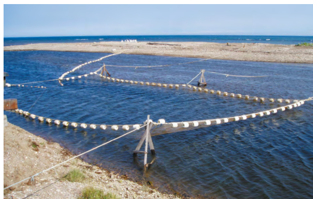
Fig. 8.5. Fish-counting barrier on the Naicha River, 2008 (photo by S. Makeev)
