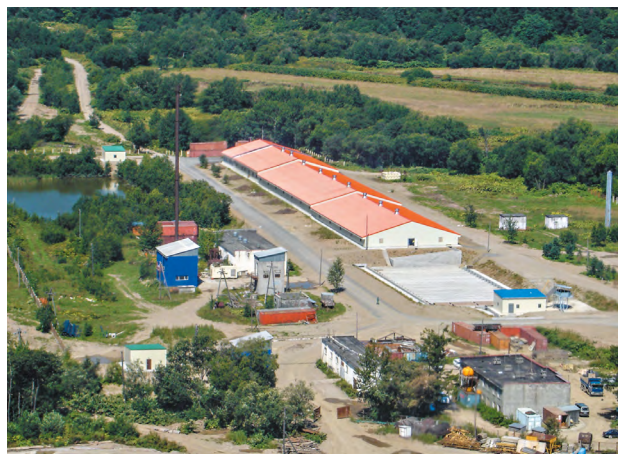
Fig. 9.4. General view of the Taranay hatchery after reconstruction
