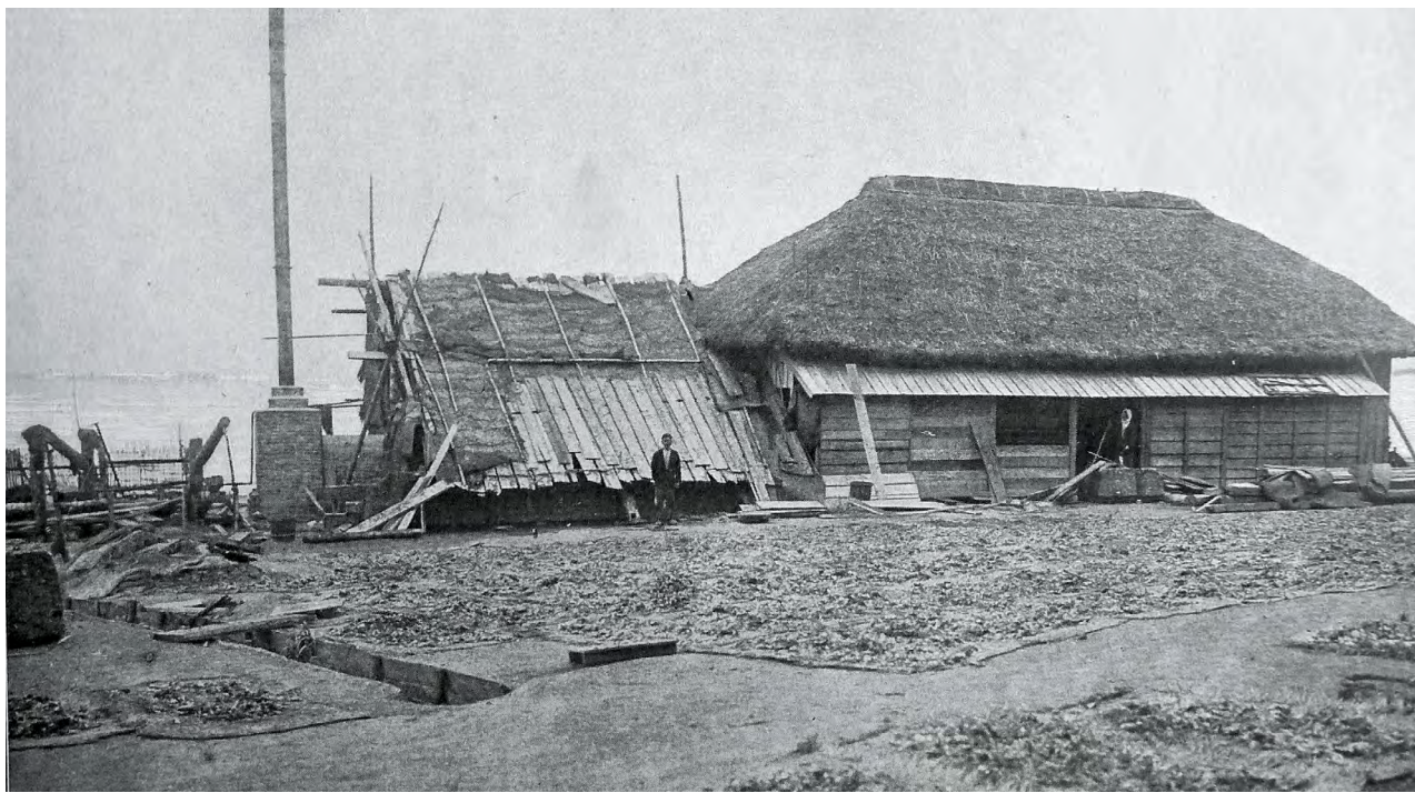
Brick oven and cabbage drying shed. 1901
