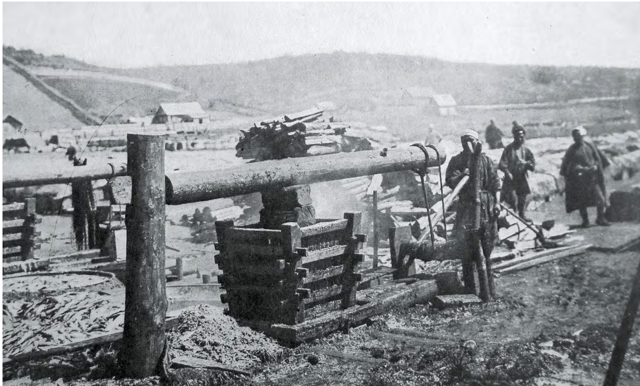
Shime-dou press for fish fertiliser. 1901
