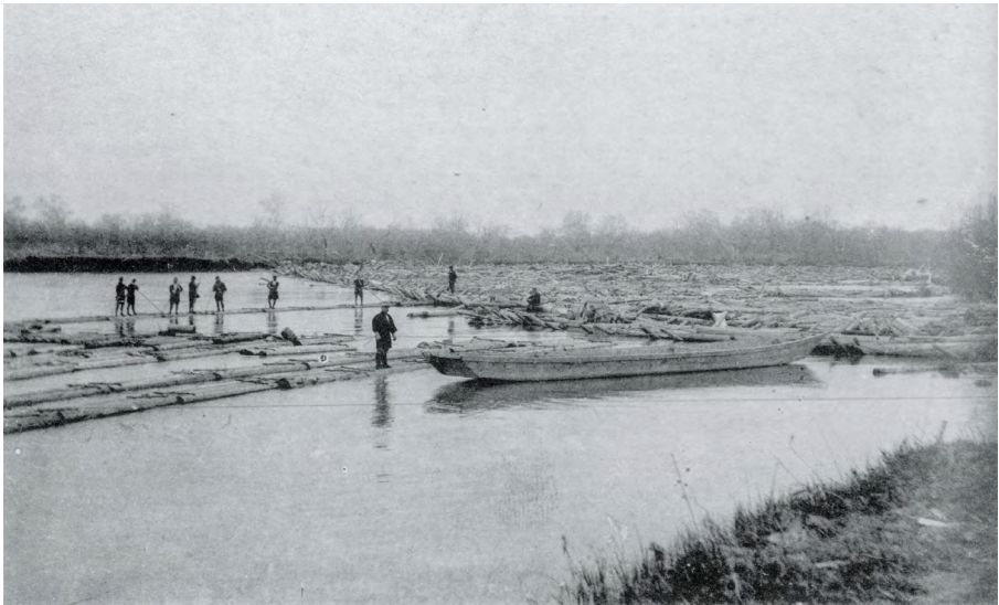
Timber rafting on the Rutaka River (now Lyutoga River). Date unknown
