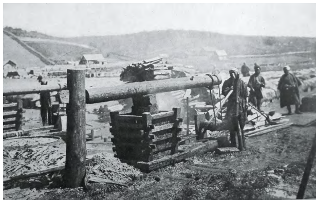
Fig. 3.5. Shime dou presses and herring cauldrons (Schmidt, 1905)
