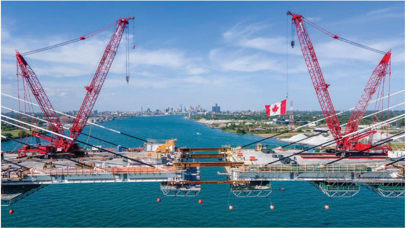
Two spans of the Gordie Howe International bridge are connected over the Detroit River during construction June 15, 2024.
