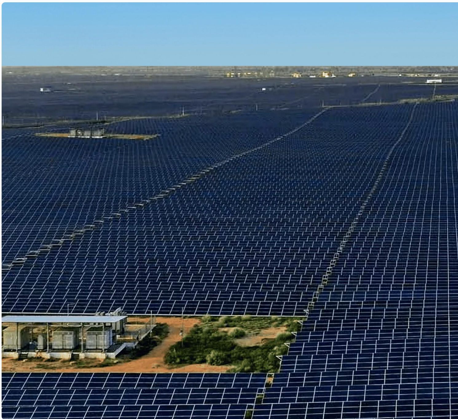
Bhadla Solar Park in Rajasthan spans nearly 14,100 acres and has an installed capacity of 2,245 MW (2.25 GW), making it one of the world's largest solar power complexes.
