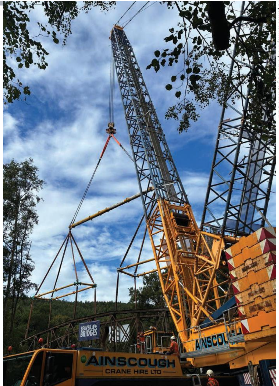
RSS delivered below-the-hook equipment for removal of the 117.5t bridge. The 10m by 3m spreader frames offered four pick points each.
