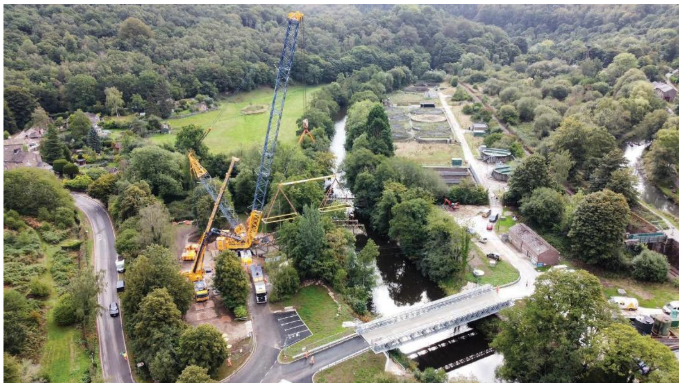
With a new bridge positioned across the River Derwent earlier this spring (foreground), Beaver Bridges was required to remove the old site access crossing.
