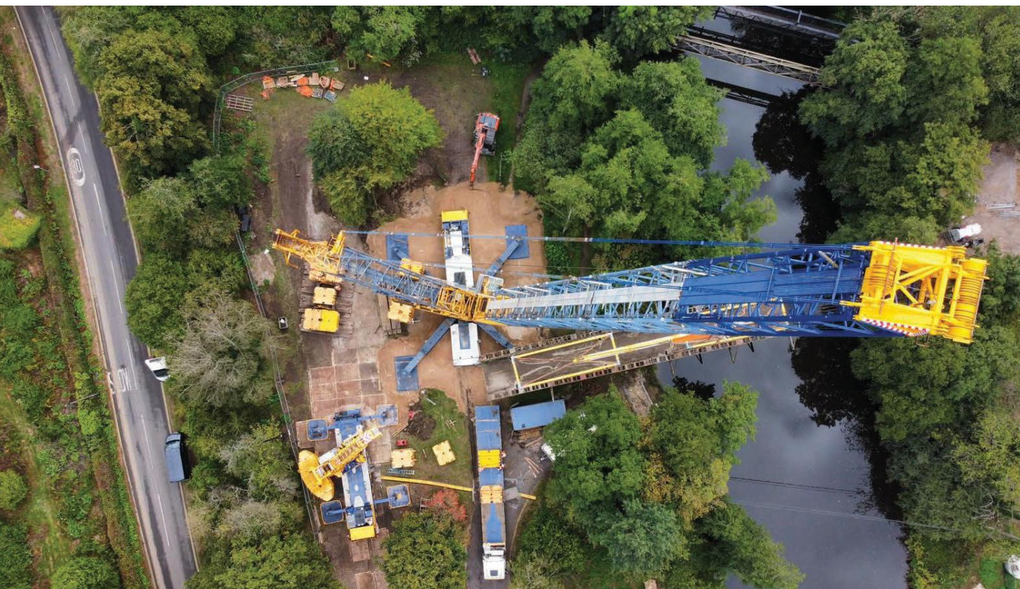
An aerial view of the Terex-Demag and Liebherr cranes at work.
