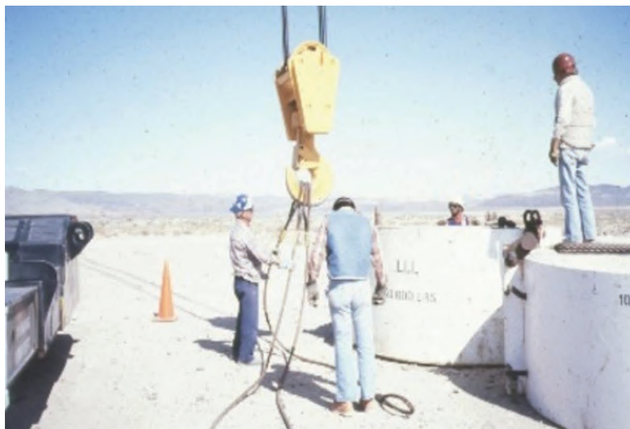
Fig. 4. Rigging is easy with proper gear, known weights, and convenient attachment points.
