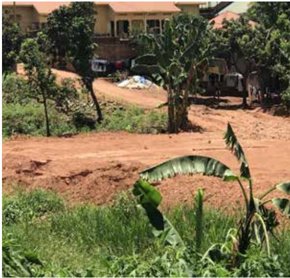
Image 7.5 House construction in the wetland
