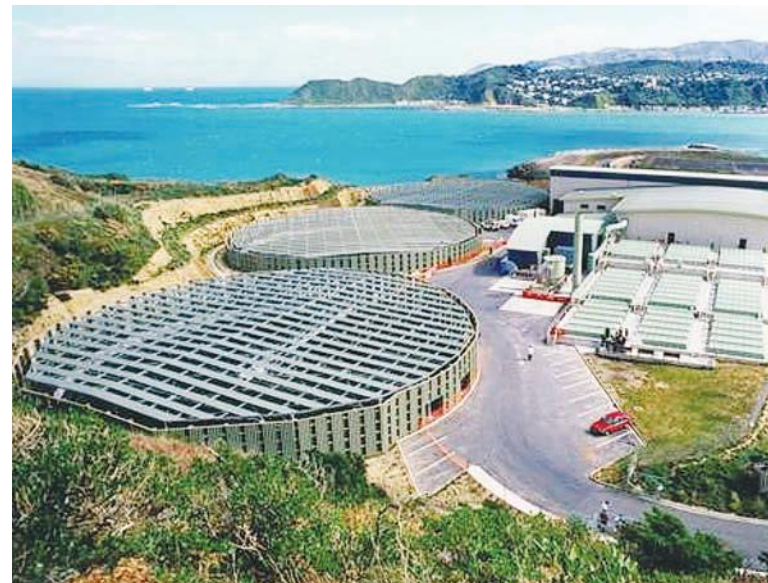
A view of the Moa Point wastewater treatment plant. Photo: Wellington City Council.
