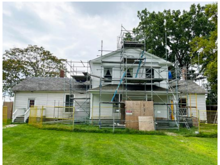
Homestead under construction. Photo courtesy of the Essex Region Conservation Foundation.
