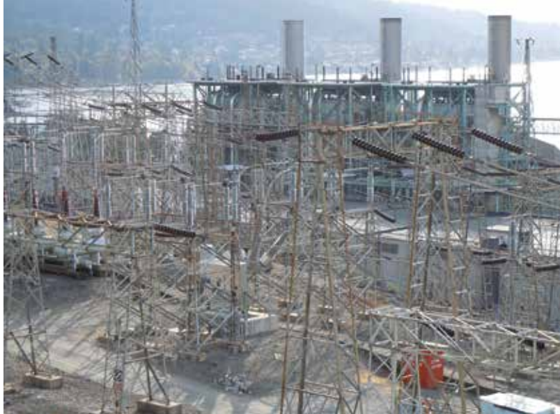
Burrard Thermal Generating Station.
