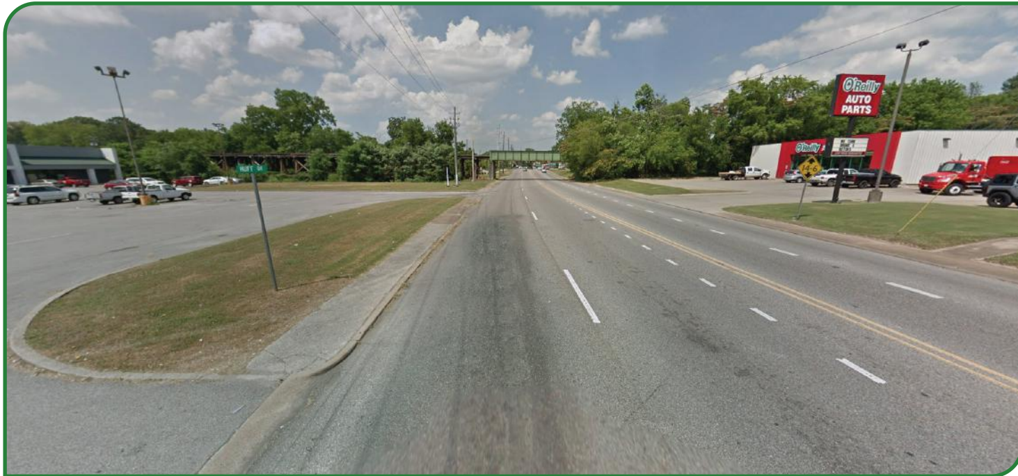
Existing Hood Ave streetscape looking north ( sidewalks/ bike lanes proposed )
