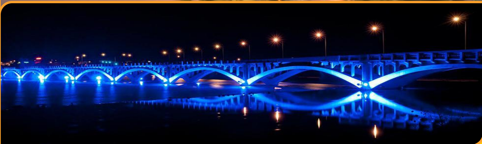
Bridge Lighting Example
