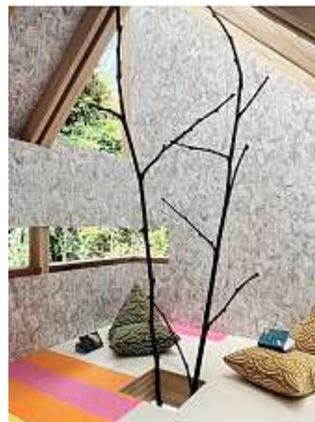
Above: SterlingOSB Zero internal linings complement the salvaged urban timber structure.
