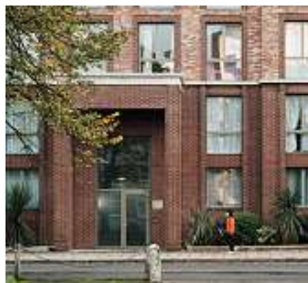
Above: At Gayton Road, Harrow, ground-floor flats are raised to offer privacy and overlooking. Common entrances are open and well-lit.
