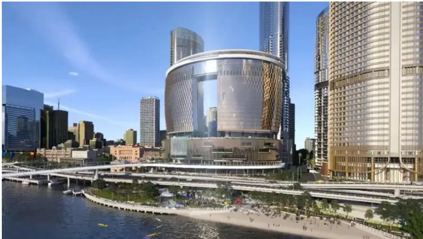
Queens Wharf Sewer, Procurement of pipes ex Germany to Brisbane, Australia, 4-month project
