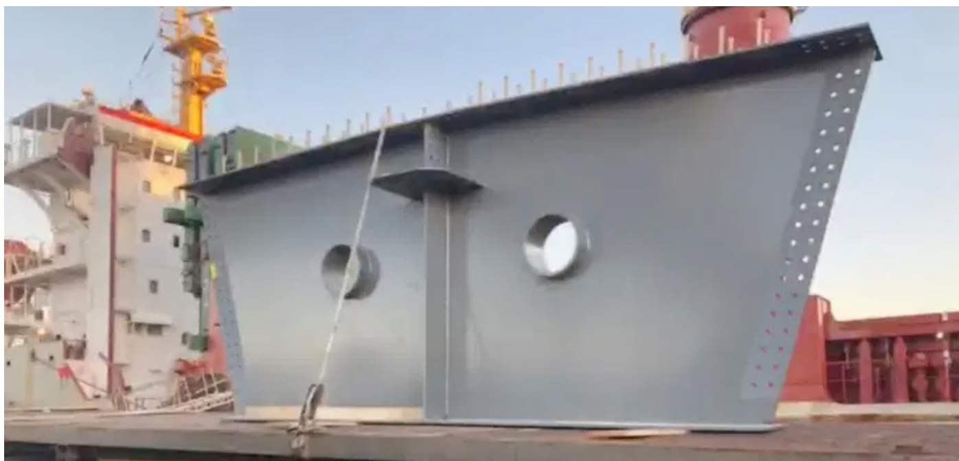
Construction Materials from Walvis Bay to Okavango Bridge Project
