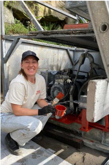
Katie painting the winch house machinery after repairs
