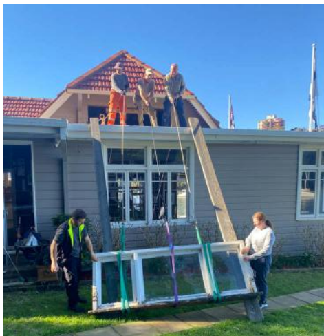
Warwick working at height repairing the window
