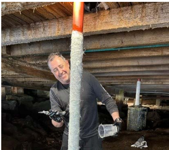
Lachlan at work on the boatshed posts
