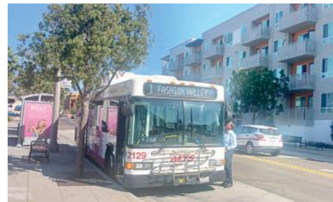
The affordable housing development at 8181 Allison Ave. in La Mesa across from a bus stop. (Photo by Drew Sitton/Times of San Diego)
