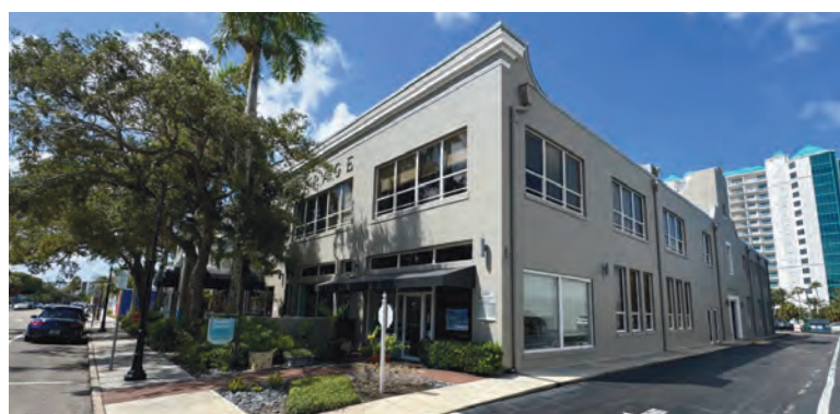
The U.S. Garage building at 330 S. Pineapple Ave., built in 1925 as the first automobile garage in Sarasota and possibly in Florida, faces demolition as a court date nears.
