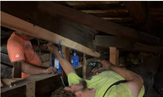
Two of the roof trusses are repaired from inside the attic.
