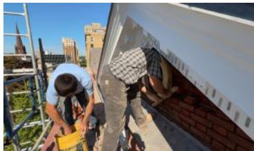
Checking the course for plumb.
