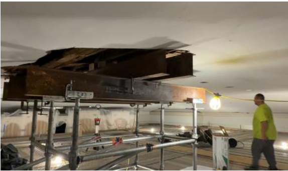
Steel and scaffolding take the weight, reaching up through the ceiling to hold the trusses while they are repaired.
