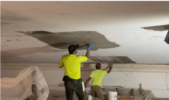
The holes left by the shoring, filled and ready for what comes next.
