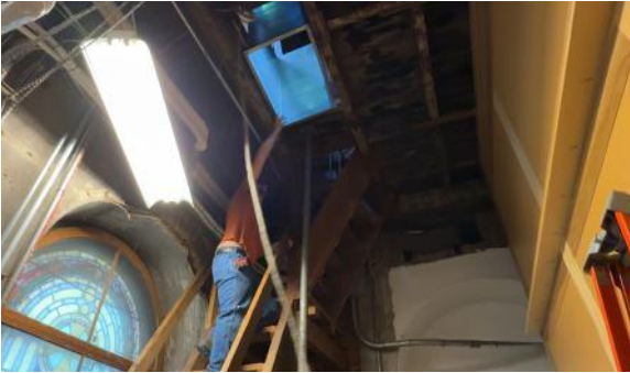
New ductwork is hoisted into the attic.
