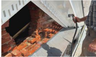
The surface must be wet for the mortar and new bricks to be set.
