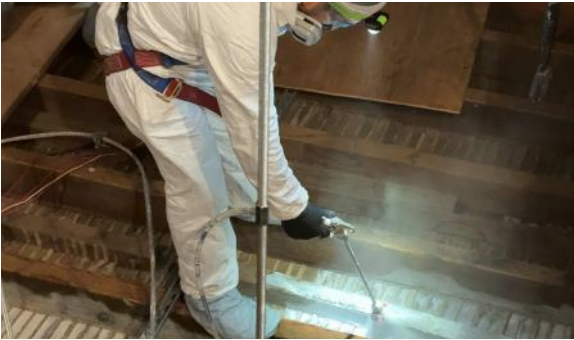
A consolidant is sprayed onto the back of the plaster to strengthen it where it sits.
