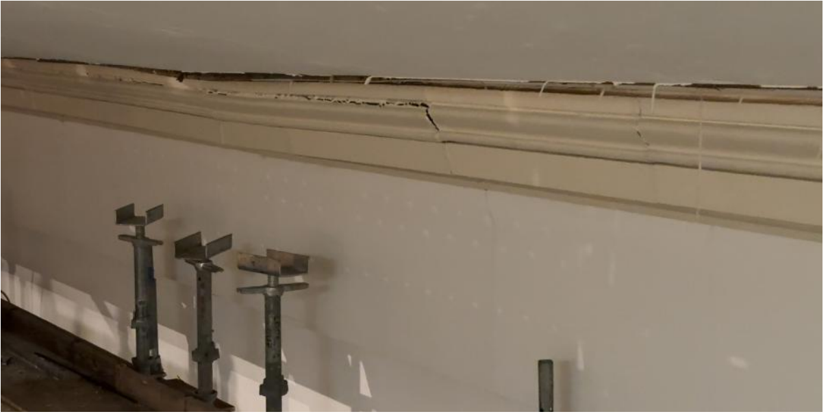
BEFORE — July 3. The crown molding on the high wall, before any work began.
