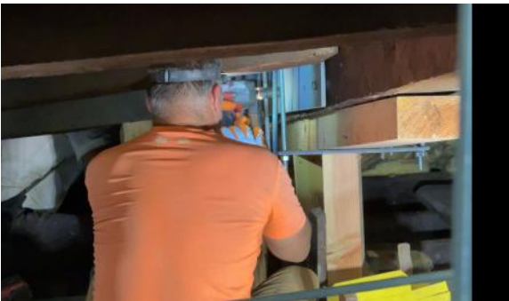
Steel gusset plates are bolted through the tie-beam joint, tying the new work to the old.
