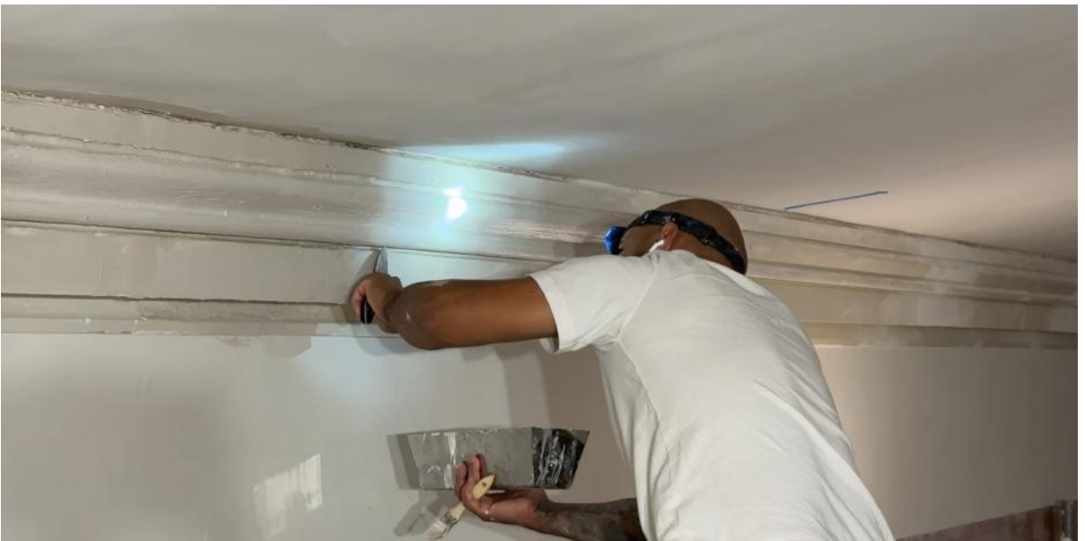
AFTER — August 24. The same run of molding, fully repaired.
