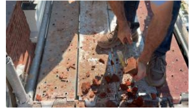
Smaller pieces are shaped with a brick hammer.
