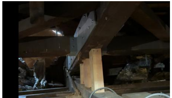
Truss repairs are complete!
