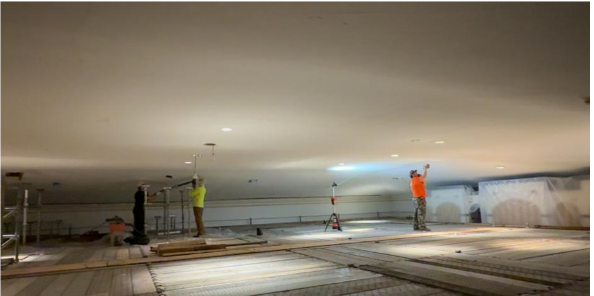
A temporary work deck goes in over the whole sanctuary, putting the crew within arm's reach of the ceiling.
