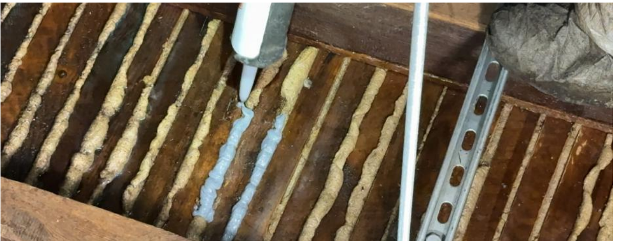
Repairing the plaster keys — the ridges of original plaster that squeezed through the lath and have gripped it ever since.
