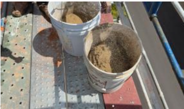
Lime mortar was used when our church was built and is the correct mortar to use now.
