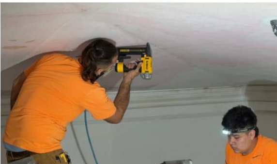
Reinforcing mesh goes on next, bridging every seam so the joints never come back as cracks.
