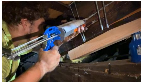
A two-part epoxy is injected into the truss cracks to bind the wood together.
