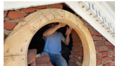
Finishing the last few pieces from the inside.
