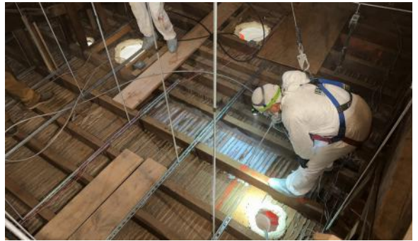
Above the ceiling, in the attic, the work begins on the original plaster — this process is known as consolidation.
