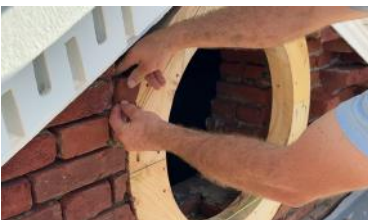
The shaped brick is set into place.
