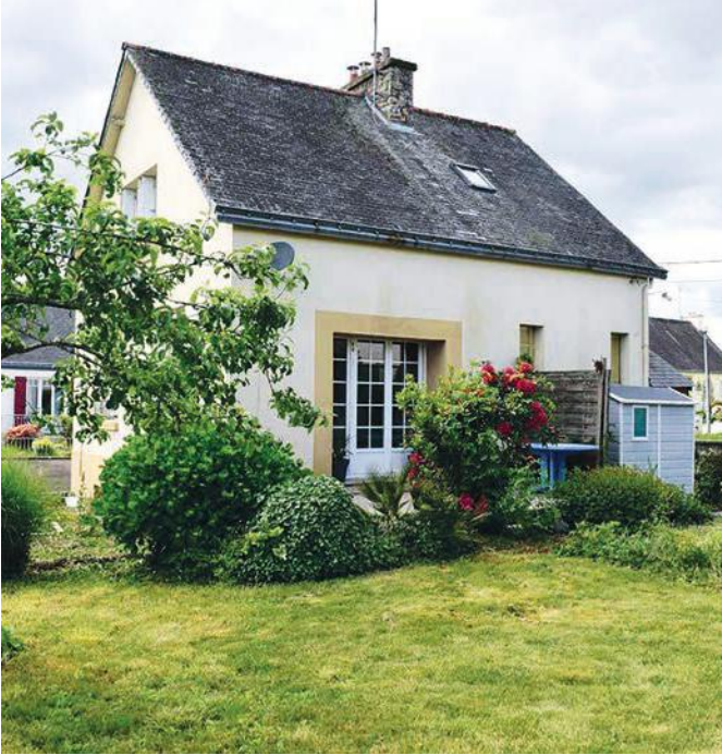
Three bedroom house with outbuildings.
