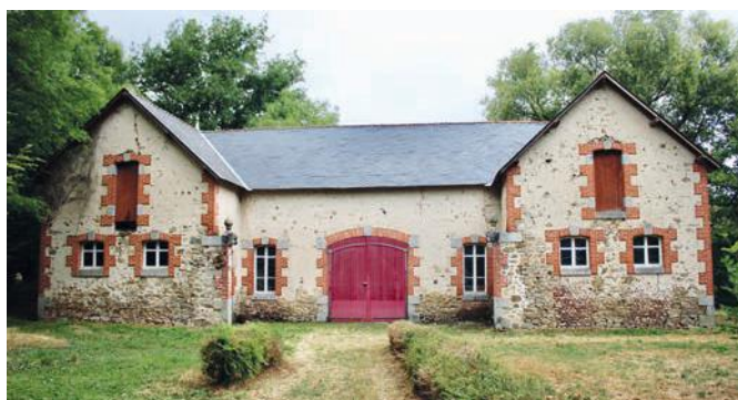
There are several outbuildings in the château's grounds adding flexibility
