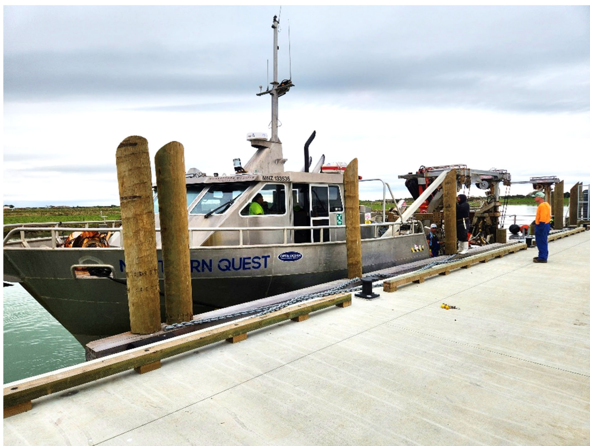
Upgrades to the Ōpōtiki wharf have been completed to accommodate the mussel boats
