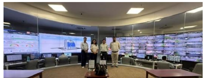
Image: Visit to the utility tunnel / district cooling facility / command centre.
