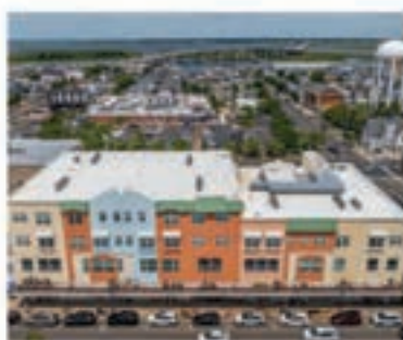
Stainton's 810 Asbury Ave
