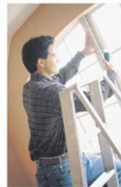
INSTALLING ENERGY-EFFICIENT WINDOWS IS ONE WAY TO REDUCE ENERGY COSTS.
