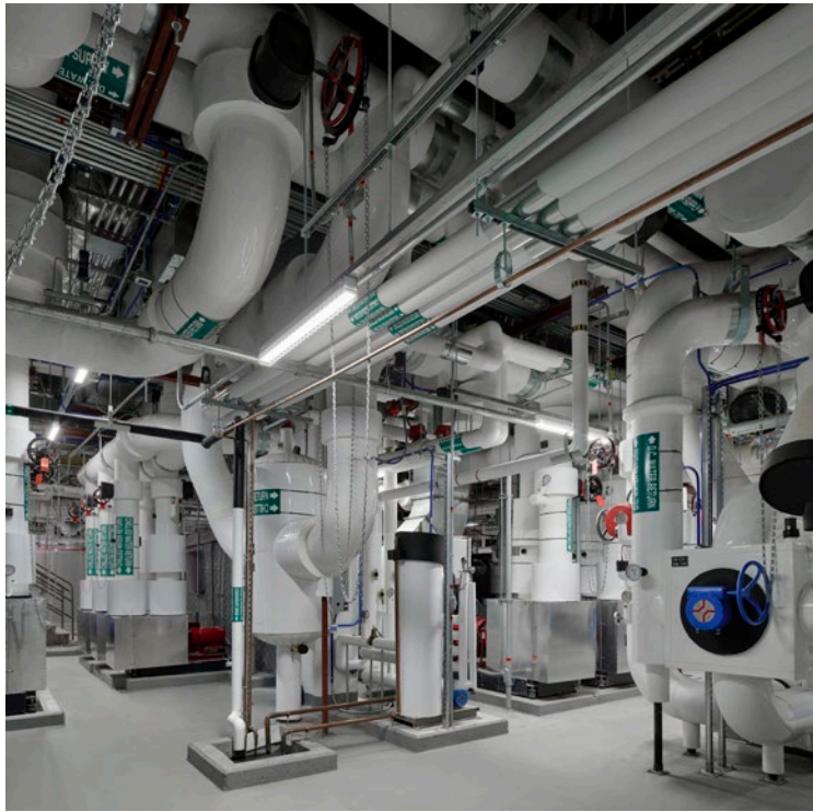
Upgraded HVAC equipment (left) serves the modernized Museum, where high-efficiency chillers and heat recovery replaced systems dating back to 1976. Electrical infrastructure (right) supports the building's controls, lighting, and life-safety systems.
