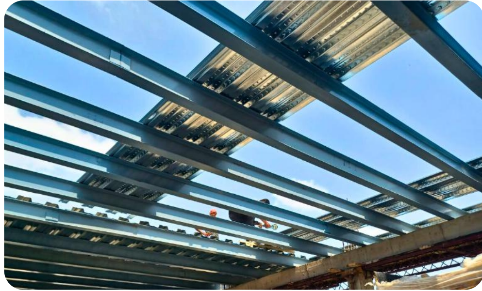
DECKING WORK MATERIALS
