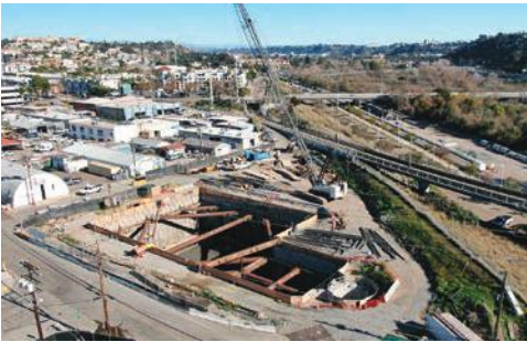
The Morena Pump Station while under construction. (Photo courtesy City of San Diego)
