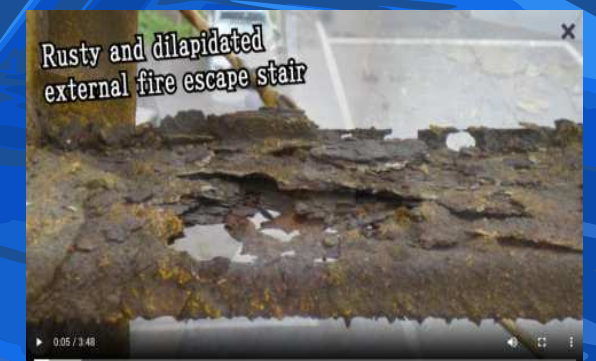
Repair of Heavily Degraded Stair case at JFE
