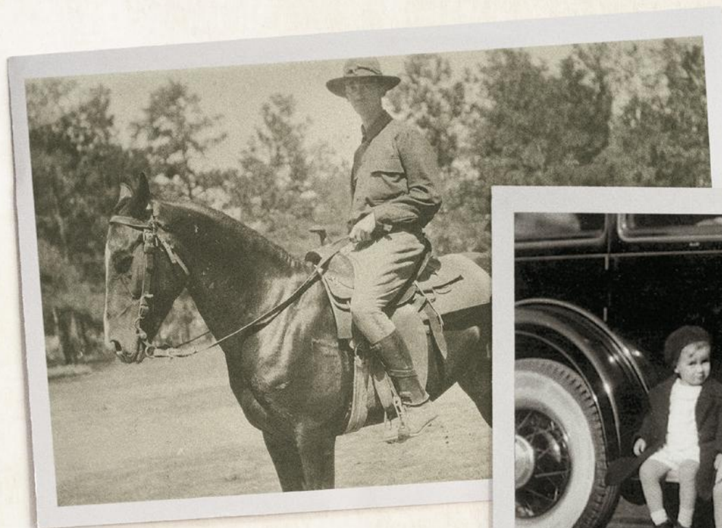
Sergeant Major (SGM) Arthur J. Gallagher, 108th Engineers, 33rd Division — the Prairie Division
